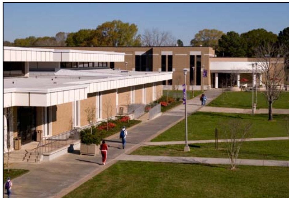
STUDENT UNION (LEFT) AND THE HEALTH TECHNOLOGY BUILDING
